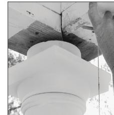
3. Slip base over top of column shaft and allow to slide to base of shaft. Slip cap over shaft and allow to rest on neck mould. Some sanding may be required.
