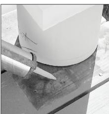
5. Apply construction adhesive in the way you would apply a caulk, around the column shaft where it contacts the floor and beam. Use your finger to press/squish the bead of adhesive into contact with those surfaces.
