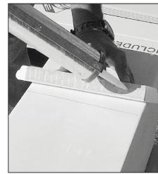
9. Mark location for supplied neck moulding. Apply construction adhesive\* and put neck mould in place.
