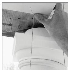
4. Put assembly in place and plumb. Make sure load is centered over column shaft and evenly distributed around the bearing surface.
