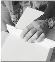
10. Pre-drill holes through neck mould into column. Screw neck mould in place prior to pre-drill and use finish nails.
